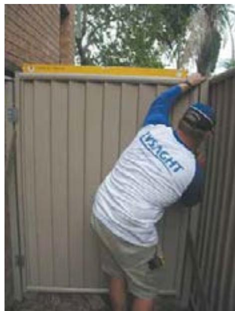
7) Hang the gate. Attach the latch, handle and drop bolt as required.
