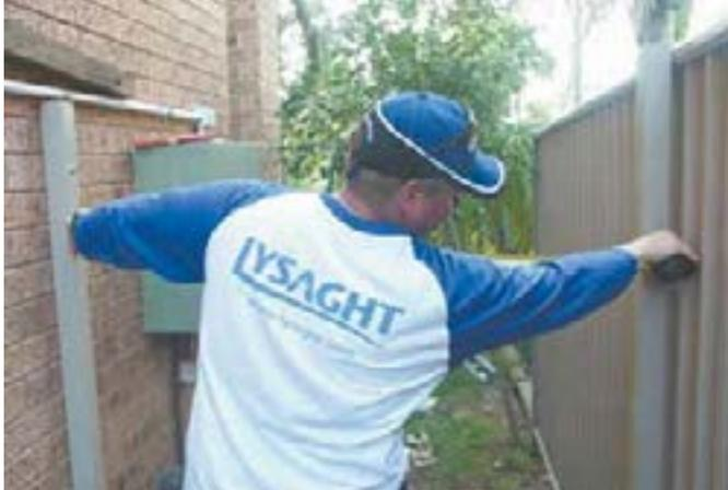
2) Measure the gap where you are going to position the gate to know where to set the posts. Measurements should allow room for the gate to swing, and for space between stiles & posts. (Recommended allowances are given on p17 of this brochure.)
