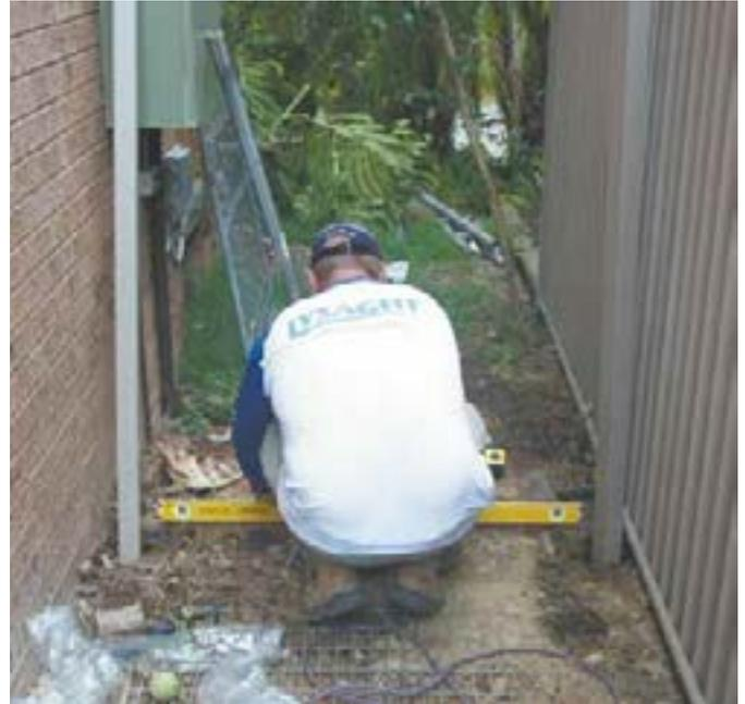
5) Use the level to double check plumb and gate positioning. Remember that a level gate swings free and easy.
