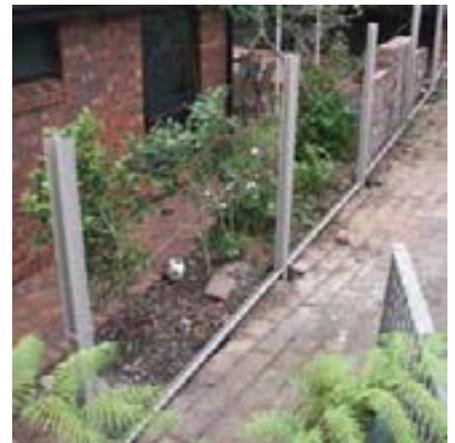
Set all the bottom rails into position ensuring a 50mm ground clearance.
