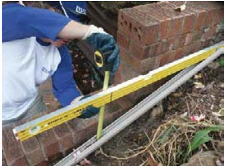
Measure the fall on the rail. This will allow you to position the top rail parallel and also to correctly cut the infill sheets.
