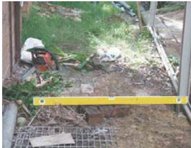
3) Set the level at the height required to swing clear of the ground. Use a measuring tape or the level to show where gate aligns with the post and mark this position (using a compatible marker or texter, not a lead pencil.)
