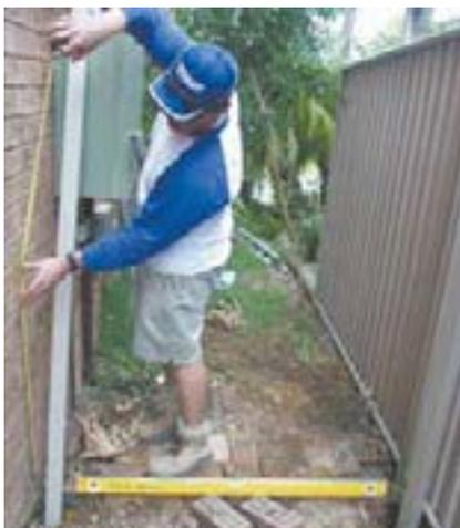
4) Set the second post so the post tops align and check it is plumb. Measure the position of gate height and mark on post.
